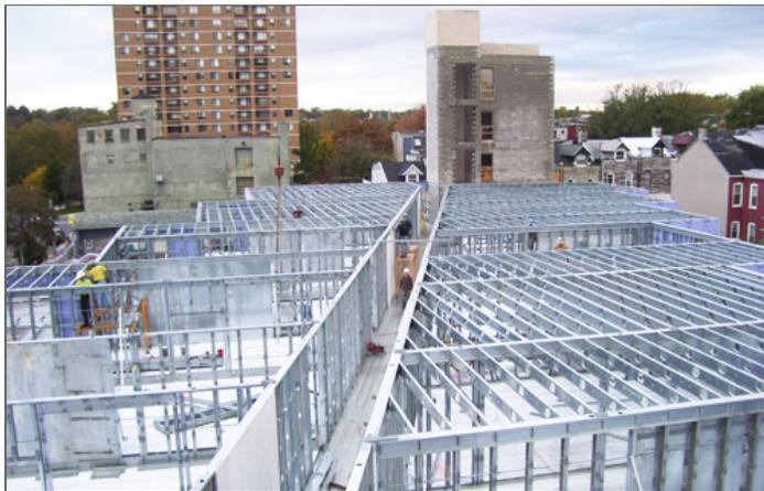
The GoggleWorks Apartments construction project in Reading uses a building process that relies on an arrangement of prefabricated steel boxes on each floor.
